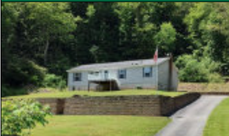
952 Marsh Creek Road, Wellsboro
