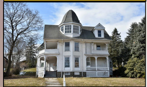
105 York Avenue, Towanda
