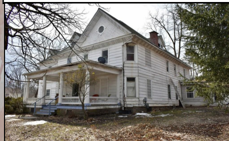
319 York Avenue, Towanda
