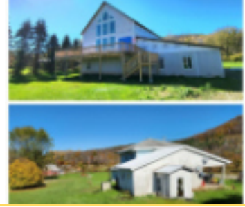
320 Hickox Road, Genesee
