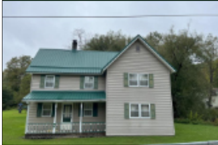
15 Bingham Center Road, Genesee
