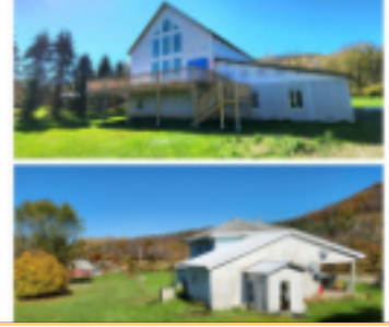
320 Hickox Road, Genesee
