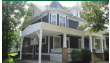
58 E. Elmira Street, Mansfield
