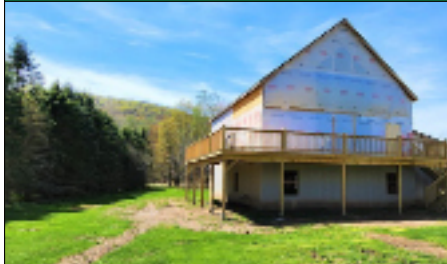
320 Hickox Road, Genesee
